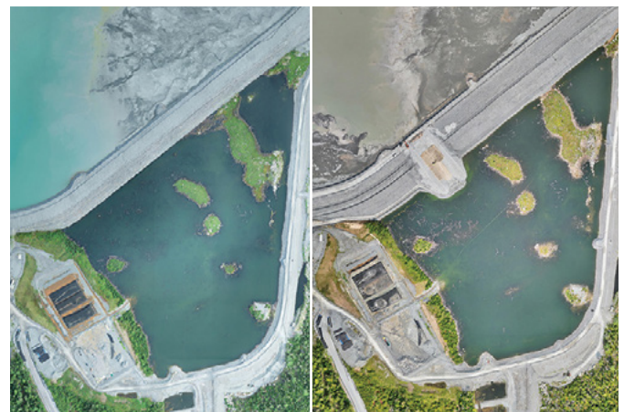
Before: Tailings management facility during operation.
