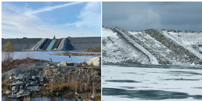
TMF spillway construction during and after.
