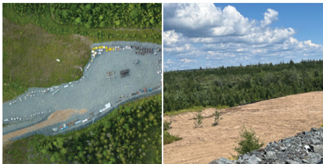
Mill laydown area before and after reclamation.
